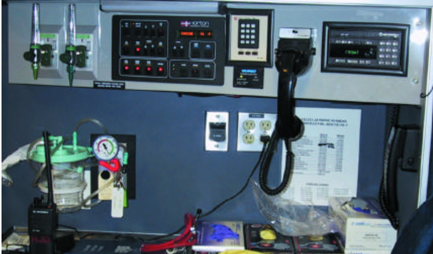
Ambulance to hospital data and voice communication equipment
